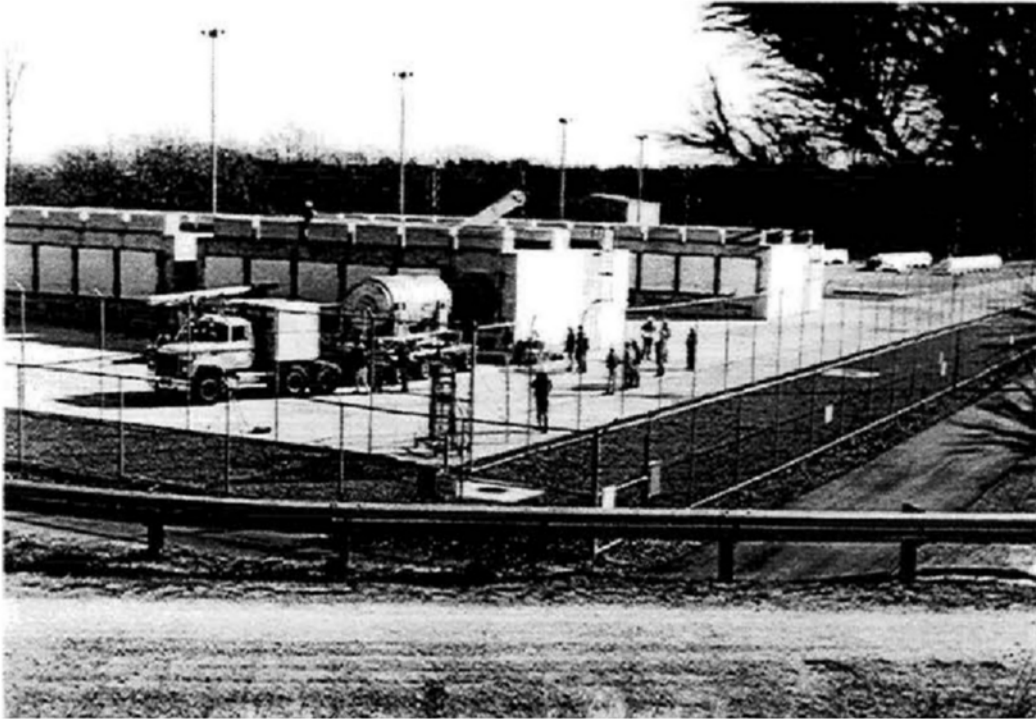
FIGURE 4.2 Photo showing a canister being loaded into a NUHOMS horizontal storage module. SOURCE: Courtesy of Transnuclear, Inc., an Areva Company.
